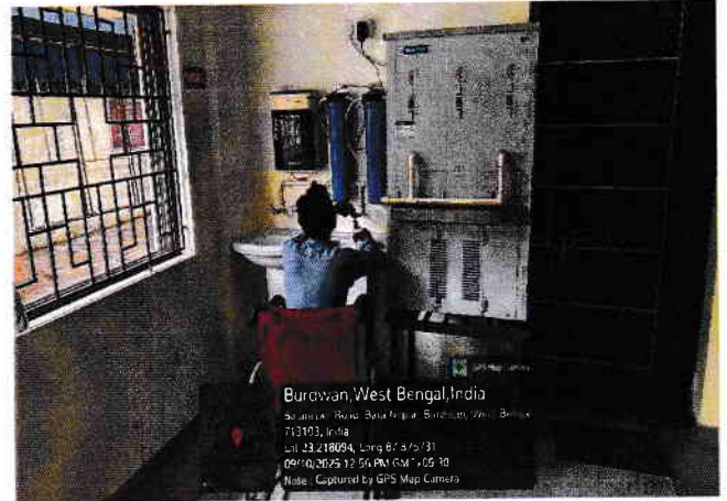
Wash basin at drinking water corner accessible for wheelchair bound Divyangjan
