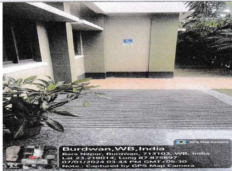
Disabled-Friendly Ramp at Academic Building
