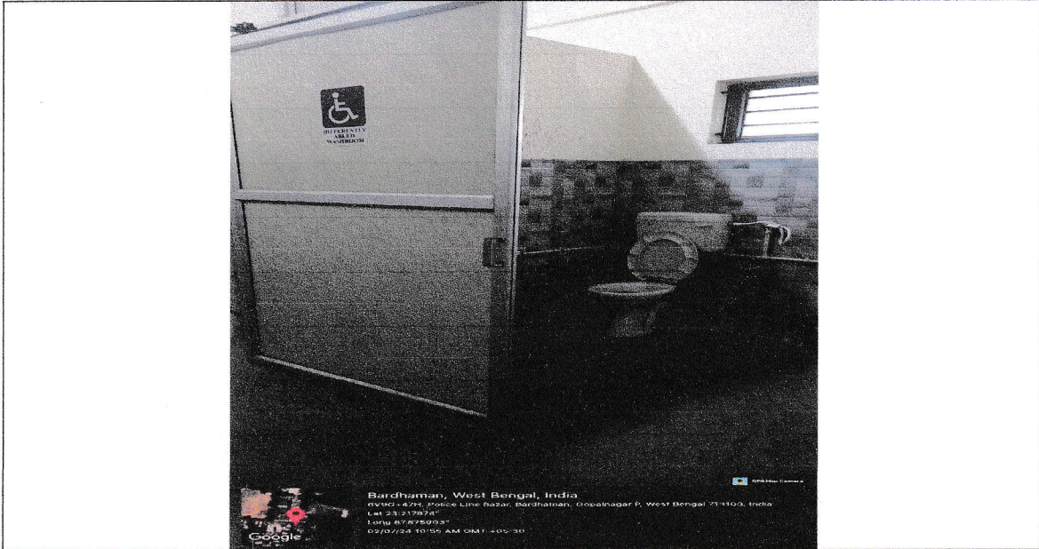
Washroom for the Differently-Abled at Academic Building
